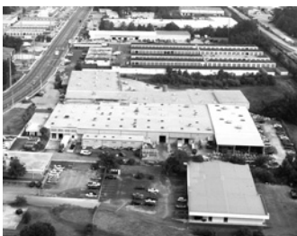
Factory in USA
